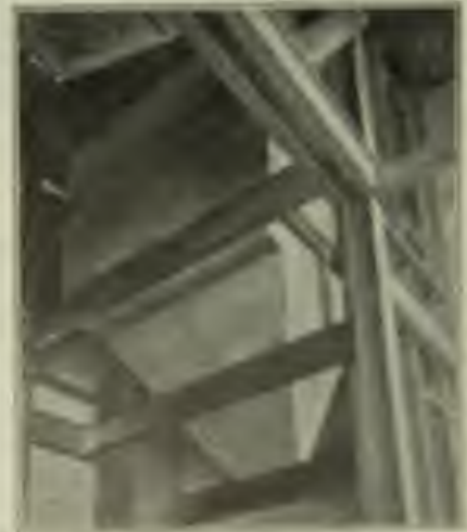
STRUCTURE FOR POWER HOUSE BUILDING
